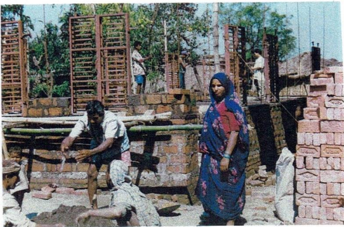
Work in progress, Community Resource Centre
