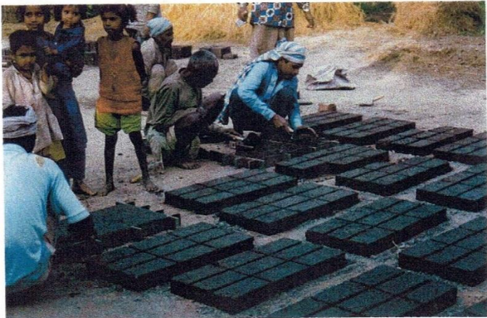
Making of lean concrete bricks
